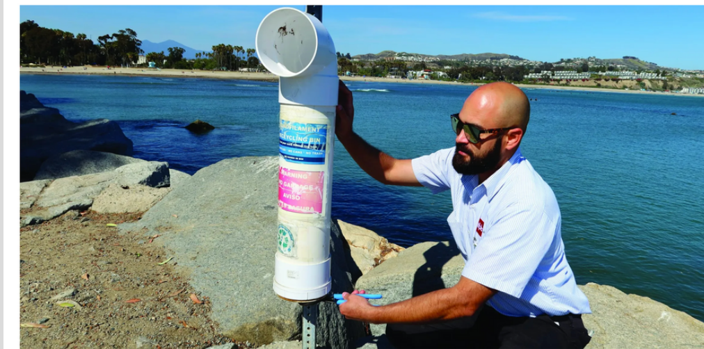
One of Dana Point Harbor Partners' environmental initiatives includes storm drain filter insert devices for trash and debris management. Photo: Courtesy of Emma Opie
